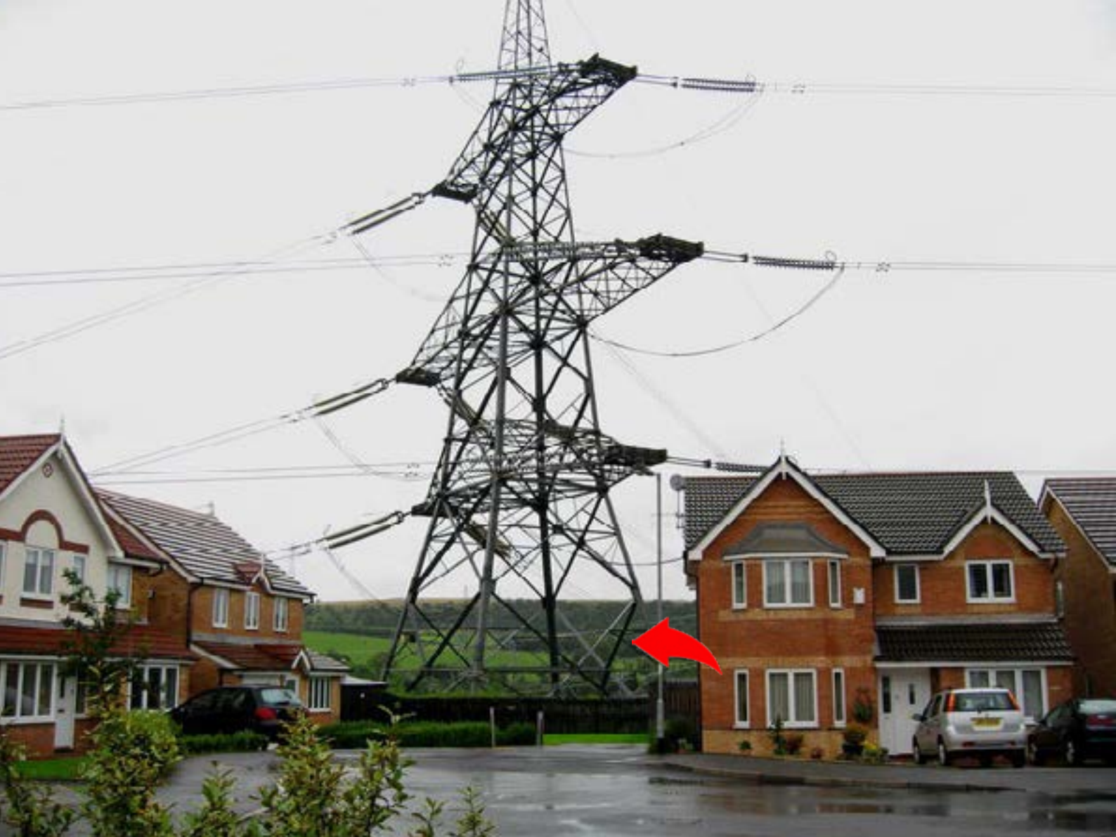
White Tiger Sha - Pylon at the right hand side of a house as shown by the red arrow.
